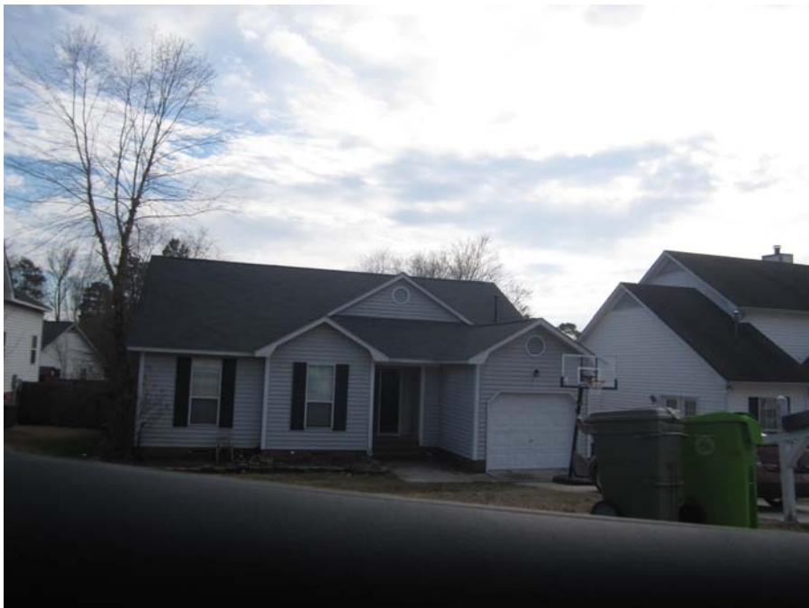
-Sample single-family home south of site
